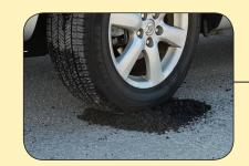
Easy compaction with a car tire or tamper.
